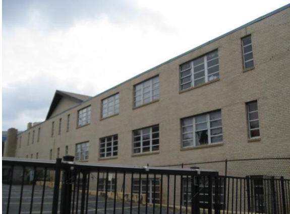
Rear of Building (Photo Taken on June 7, 2013)
