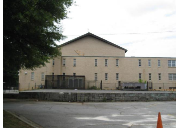
Rear of Building (Photo Taken on June 7, 2013)
