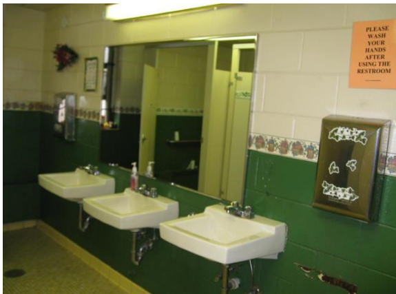
Typical Restroom Area (Photo Taken on June 7, 2013)
